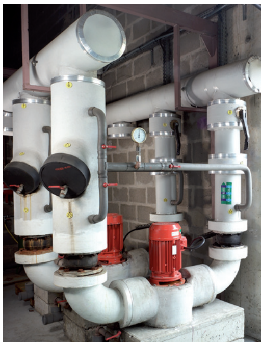
Example of using the Altistart 22 soft start/soft stop unit in a pumping application
