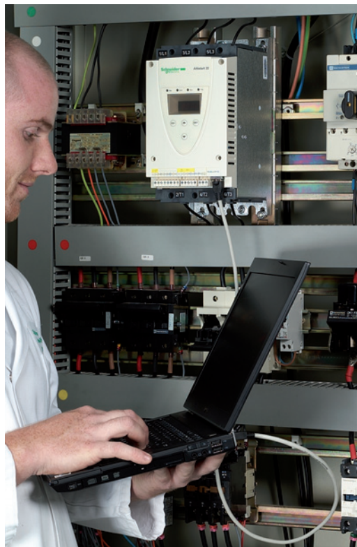
Testing and start-up of the ATS 22 soft start/soft stop unit using SoMove setup software
